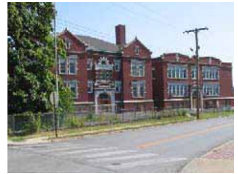
VACANT SCHOOL BUILDING
