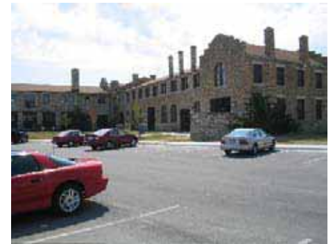
THE GENERAL OPERATING PLANT
