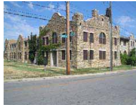
THE GENERAL OPERATING PLANT
