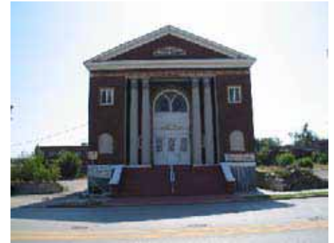
ABANDON CHURCH BUILDING
