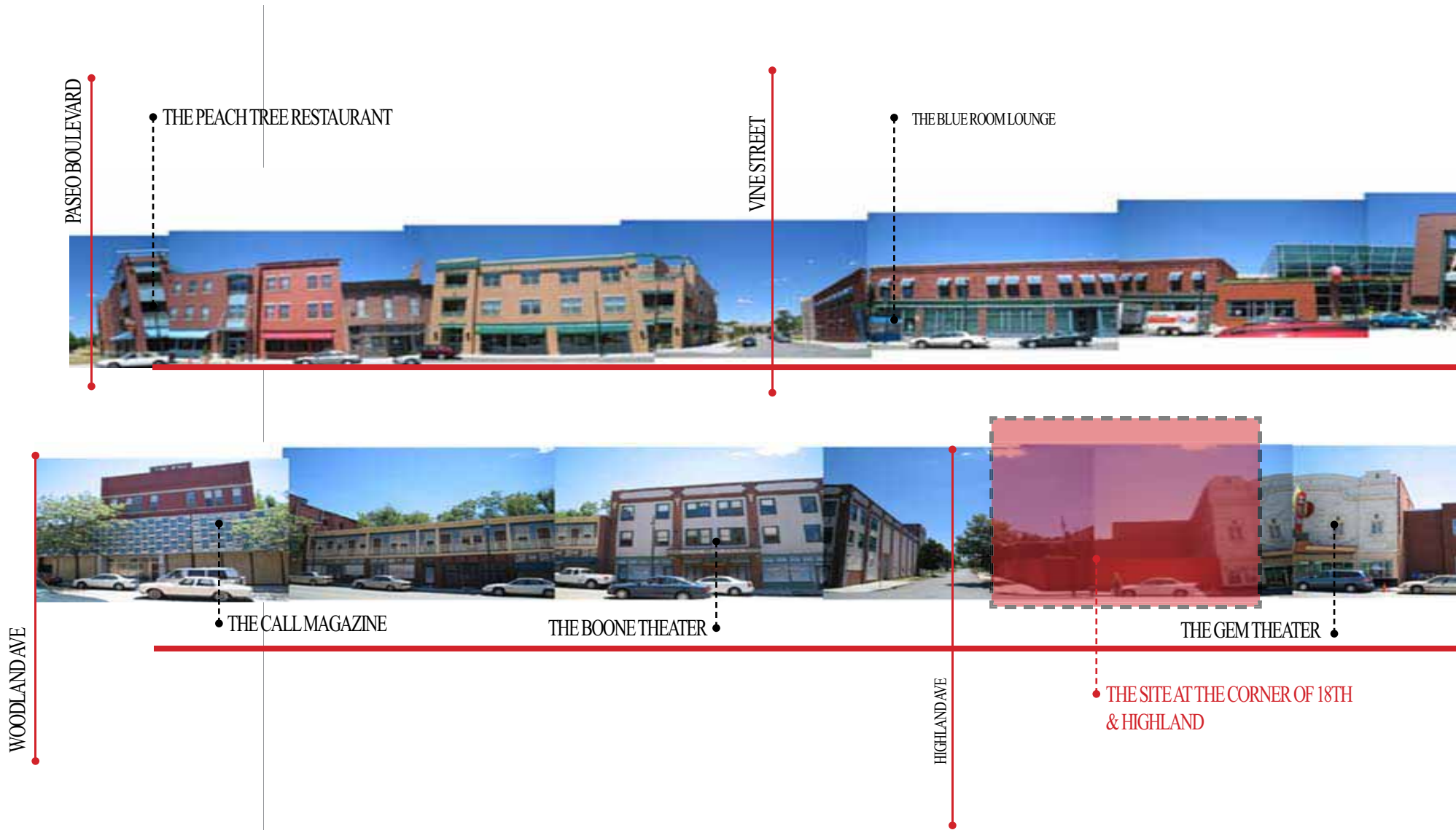
FIG. 3.6 SITE/ STREET PHOTO NORTH & SOUTH
